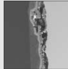
Fig 7I - Coating I on rust
