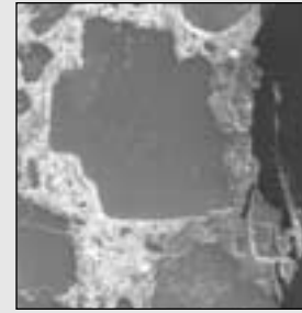
Fig 3 - Coatings on green concrete and paste; aggregate is fractured from blasting
